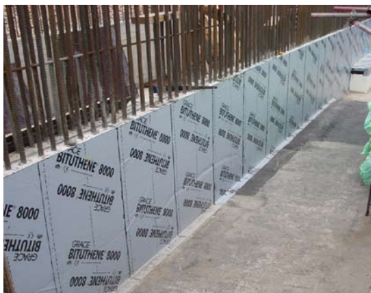
Application of Bituthene 8000
